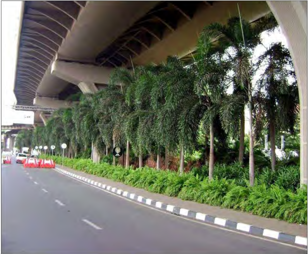
Exit road landscape towards elevated road, CSMIA
